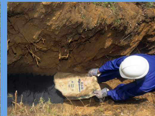
SPREAD INTO PLACE
