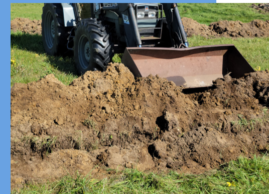
BACKFILL* Add water if in dry climate
