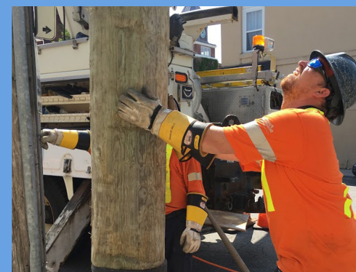
LOWER INTO PLACE
