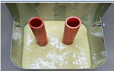
Fill gaps with FST-BP or PFP
