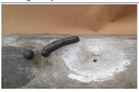
7. After approximately 2 minutes of kneading/mixing, material will feel warm to the hand. Roll the Putty into a rope about ¼ inch (6 mm) thick or a small ball the size of a pea ¼ inch (6 mm) for pin hole leaks. Apply the putty over leak and push putty so it covers about ½ inch (13 mm) from all points of the leak area with a thickness of approximately ½ inch (3 mm).
