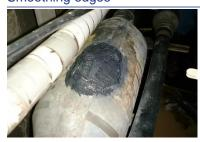
12. If the cable has been moved out of its normal position for repair, the best time to reposition is immediately after you have applied the sealant. Don't wait for full cure. The repair will be most effective if movement is limited.
