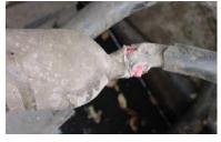
1. Cable should be as dry as possible. Pump standing water out of manhole if water is present. Wear nitrile gloves (provided) and safety glasses. Clean and dry the area around the leak with a dry rag.
